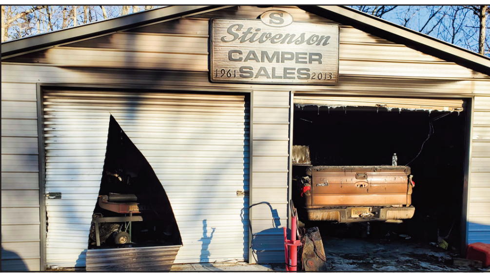
Firefighters had to cut into this metal garage building at a property off Fortenberry Road, where they battled both a structure fire and a wildland fire Feb. 14. Photo/Facebook
